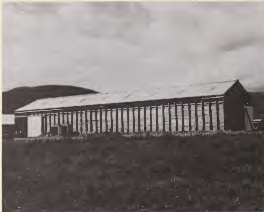
Chris DeWitt's covered-in horizontal silo measures 160 feet long and 45 feet wide. Filled to a depth of 12 feet it has capacity for 1700 tons of silage.
